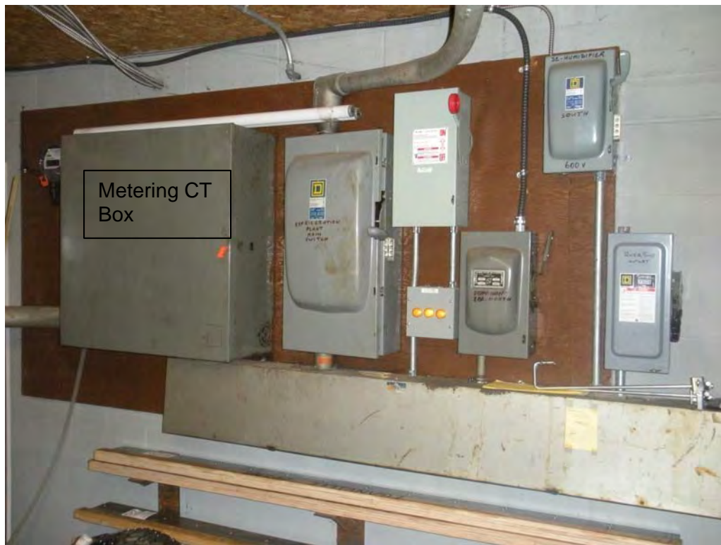
PHOTOGRAPH NO. E2 – Splitter through 600 V, 3 Phase
