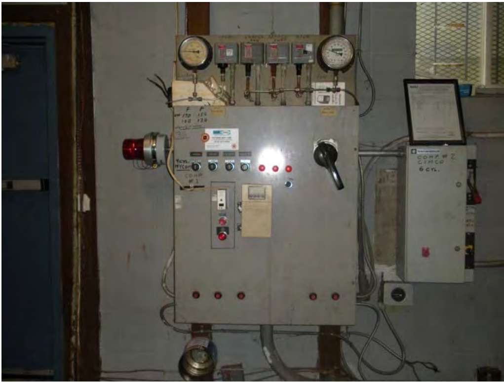
PHOTOGRAPH NO. E6 – CIMCO Refrigeration Control Panel.
