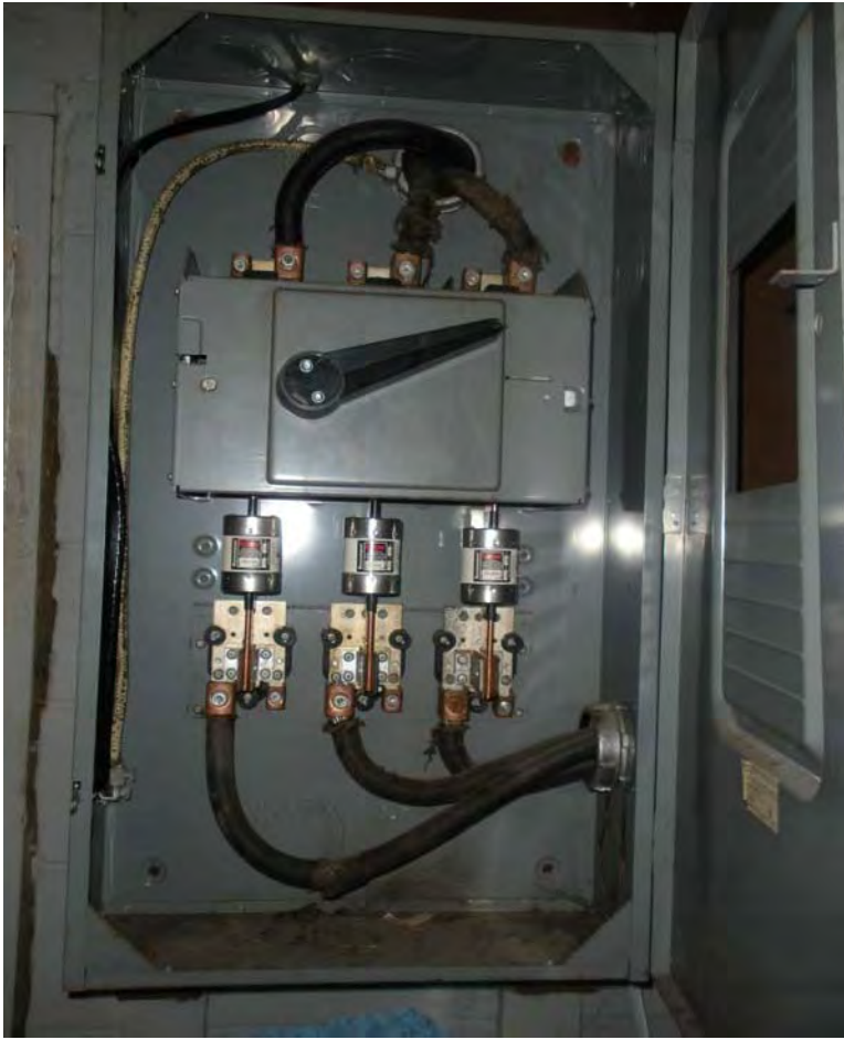
PHOTOGRAPH NO. E3 – Inside the 400 Amp, 600 V Disconnect Switch.
