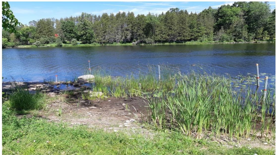
Photo 6: Boat launch helical piles
