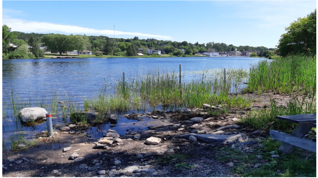
Photo 5: Boat launch helical piles
