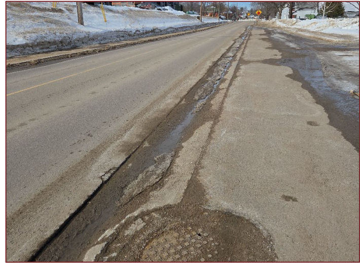
Photograph 6 – Looking west along Queen Street with a manhole cover in view.
