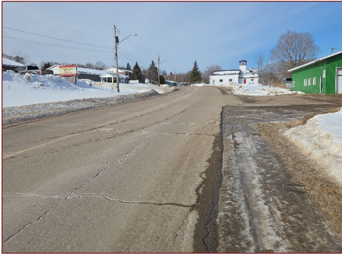
Photograph 1 – Looking west along John Street.
