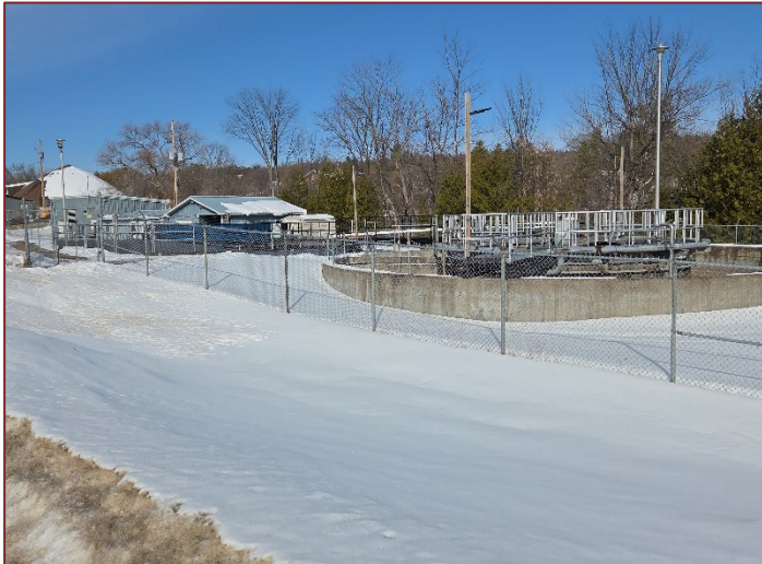
Photograph 7 – Looking north at a wastewater treatment facility located adjacent to the Project Area.
