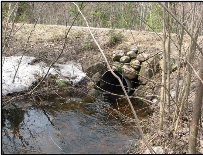
Photo 10. Watercourse identified as #121 (photo April 15, 08)
