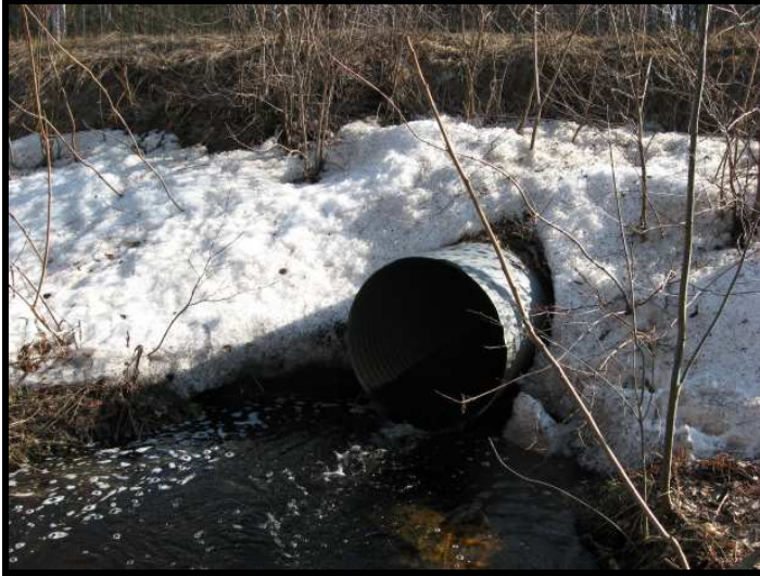
Photo 9 Watercourse identified as #78 (photo April 15, 08)
